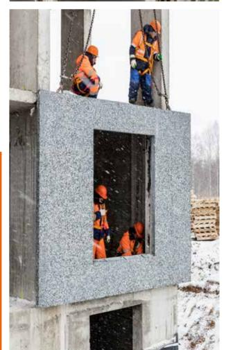
Weighing under 30 kilos, the FaMe Lite aluminum 2 x 1 m door mold is lighter than any other typical solution on the market. It is easy to move around manually.
